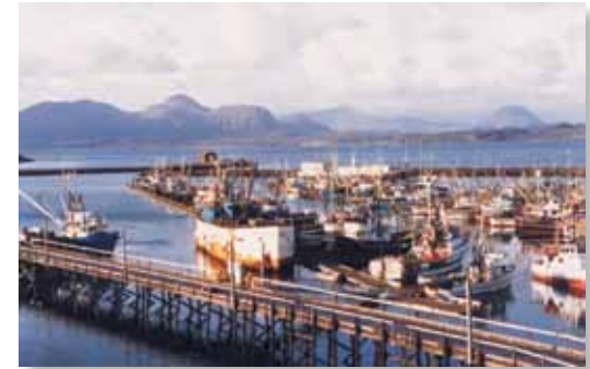
Sand Point dock—State of Alaska © Community Photo Library
