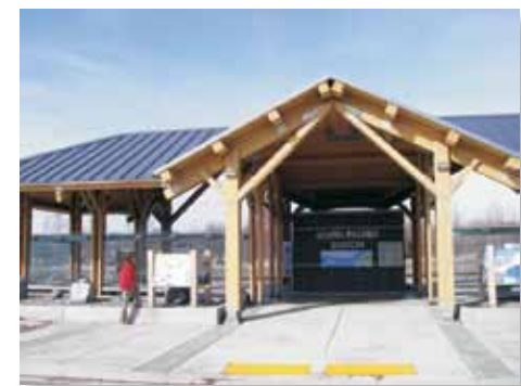
Figure 9. South Palmer Station Structure
